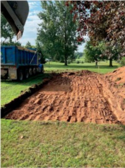
Excavated rockbed with scratch
