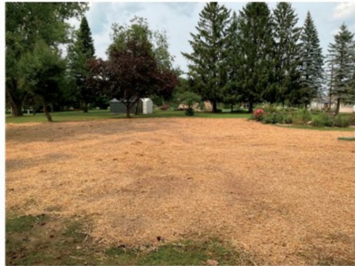
Final grade, seed, and cover over the new pressure bed
