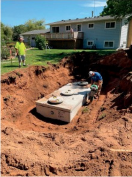
Packing around the tank prevents the soil from settling.
