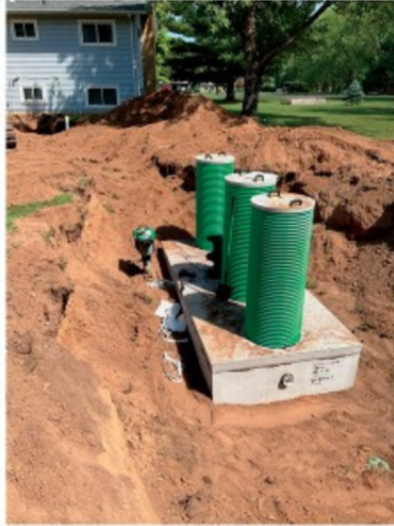
Risers are added to make the tank accessible.
